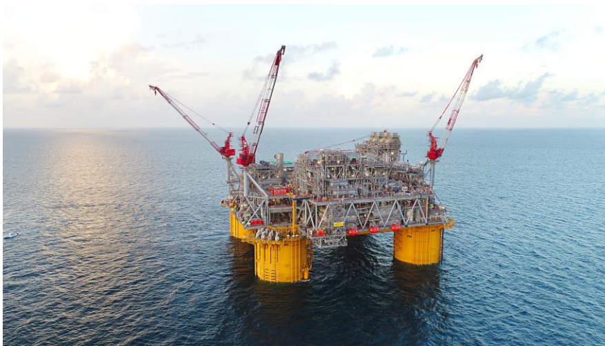
Shell Appomattox deep-water asset in the Gulf of Mexico © Photographic Services, Shell, Allison Smith
